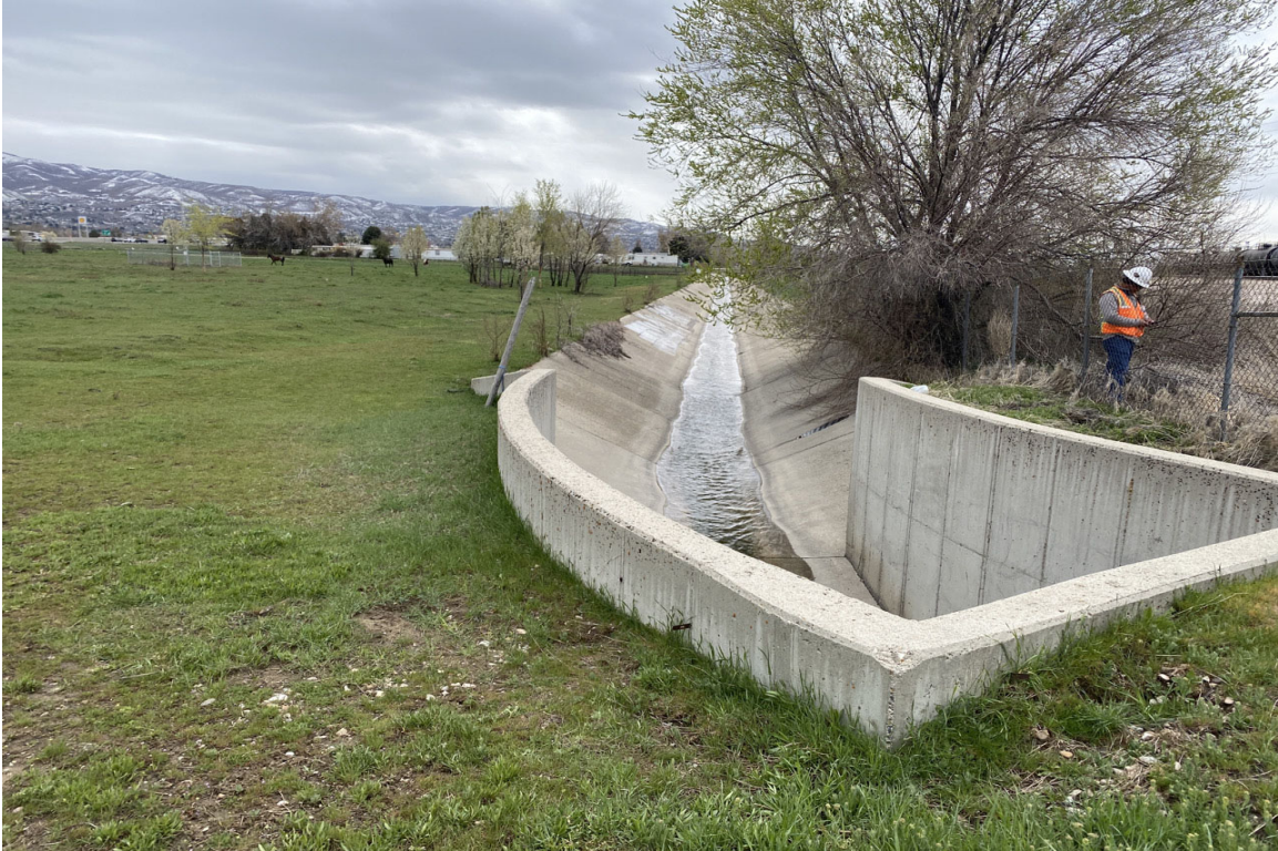
PP-WC-04, looking south at Mill Creek canal
